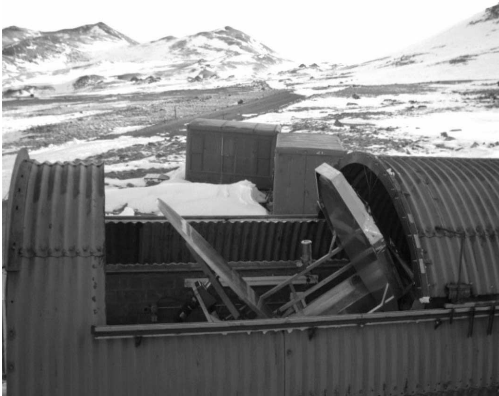
FIG. 17.—BEAST telescope housed within the modified storage garage at Barcroft Station near White Mountain, California. A section of the roof was cut from the building and placed on rollers to protect the telescope during poor weather conditions. [See the electronic edition of the Supplement for a color version of this figure.]
